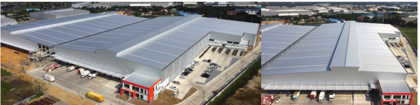
WHA KPN Building H, Bangna Km. 23: T-65DS (Double Seam System), Steel metal sheet
