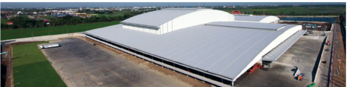
Boonrawd Brewery Distribution Center, Wangnoi, Ayutthaya: T-65DS (Double Seam System), Steel metal sheet
