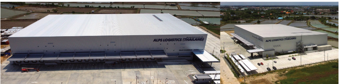
ALPS Logistics (Thailand), Bangna Km. 36: T-65DS (Double Seam System) & T-30PU (Bolt System), Steel metal sheet
