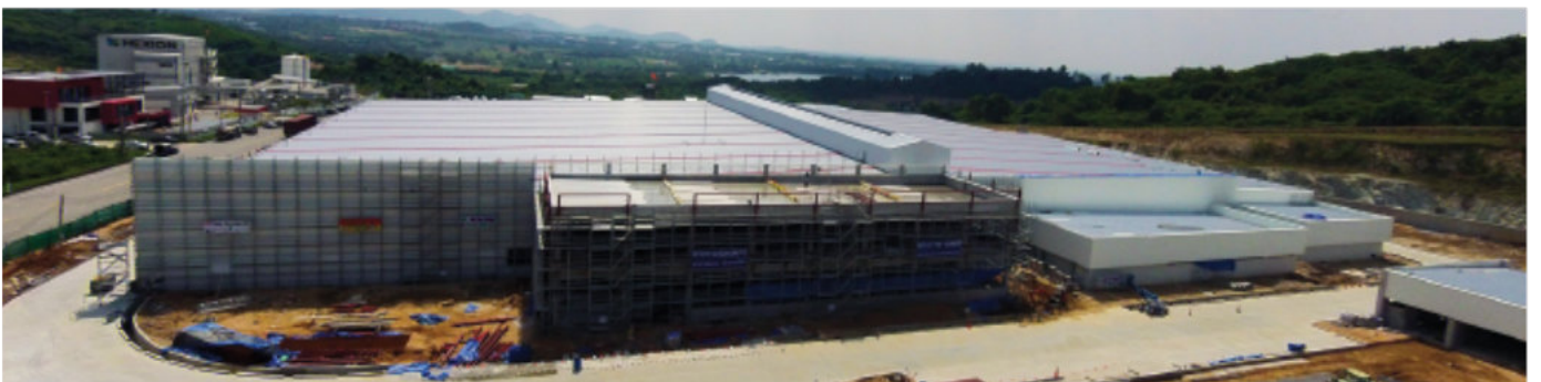
Univance (Thailand) Co., Ltd., Pingthong 2, Chonburi: T-115DS (Double Seam System), Steel metal sheet
