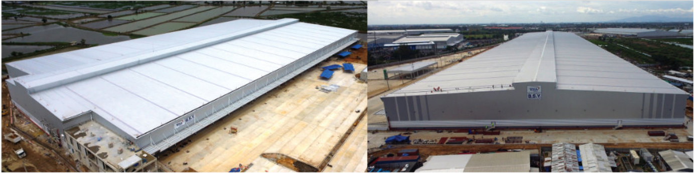
WHA E-Commerce Park (Building A), Bangna Km. 36: T-65DS (Double Seam System), Steel metal sheet
