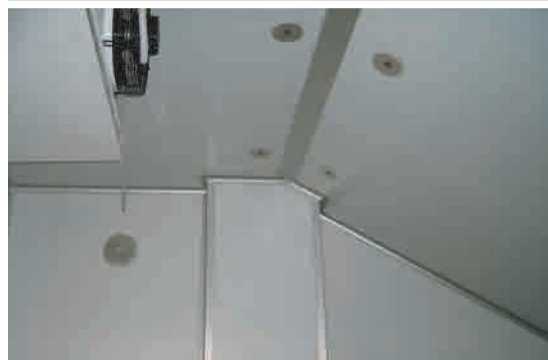
Cold Storage Room
