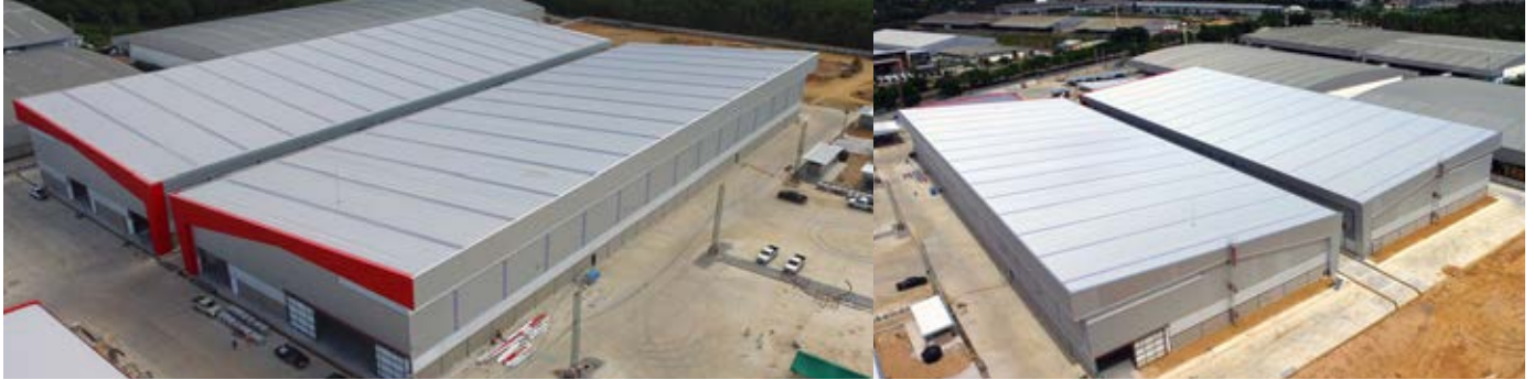
RCK 4.0, Rayong: T-65DS (Double Seam System), Steel metal sheet
