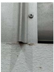
Fixed by screw on to purlin
