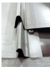
Install next panel on top of the screw to prevent the exposure directly to the weather
